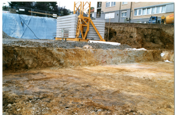
Figure 6. The occurrence in the excavations near the Hôpital Saint-Nicolas in Eupen of a 25 to 30 m wide clay zone within Givetian limestones, marking the passing of the Stadtgraben Fault (see Fig. 4). Note in the left part the steeply dipping black layers, possibly representing the geometry of the original limestones.
