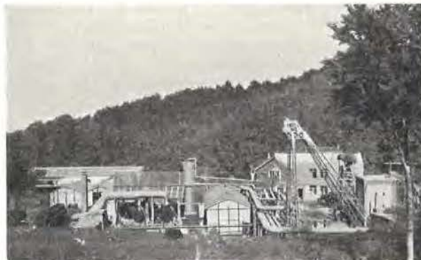
Fig. 6. — Installations de surface.
