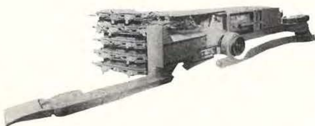
Fig. 71. — Dauerwühler ou Continuous Miner Eickhoff.
