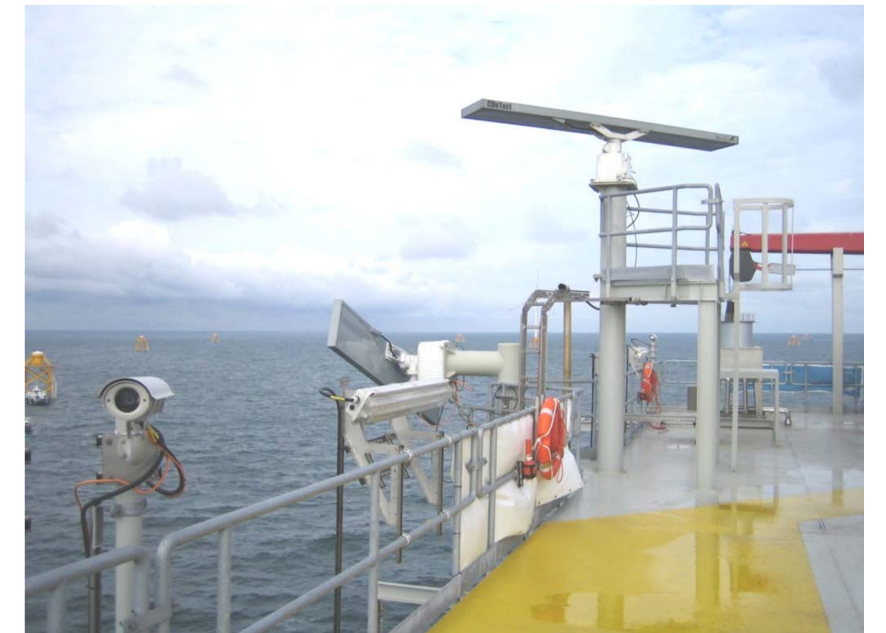
MERLIN bird radar on the offshore platform in the C-Power wind farm
