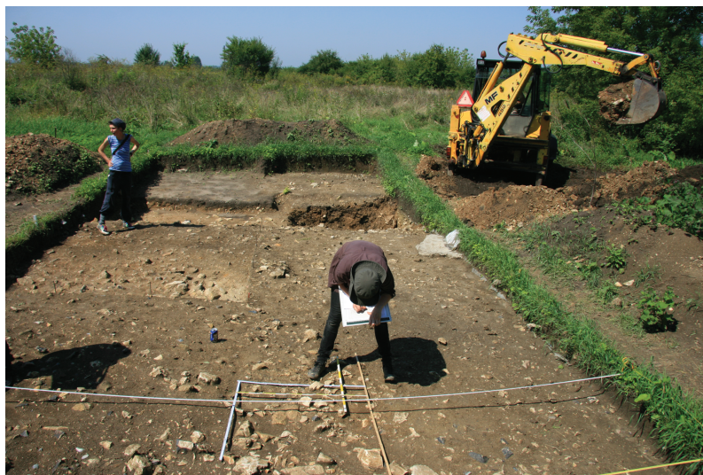
Fig. 8 – Wierzbica, Radom district (Poland). 'Zełe' mine. View from E onto cutting from 2014. in the advanced phase of the excavations. In the foreground Shaft 82 is being drawn, while a digger is uncovering old cutting I/1980, supervised by Dr Dagmara H. Werra. Photo by J. Lech.
