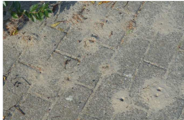
Fig. 5. Characteristic nest entrances of Tapinoma sp. MAGN resembling small volcanoes were found along the footpath of the Perziekenlaan in Ostend.
