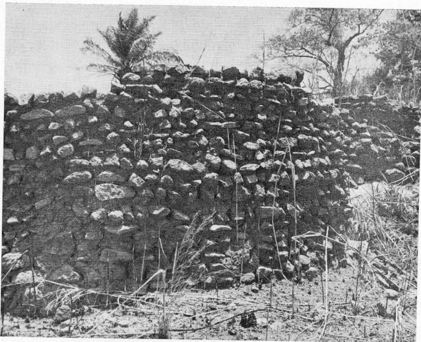
FIG. 6. — Close-up of remains of stone-walled house at old mountaintop village of Yagala.
